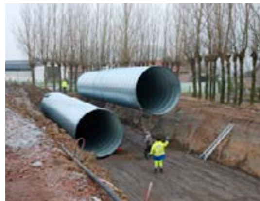
Installation of a rainwater tank
