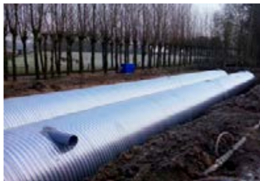
Installation of a rainwater tank
