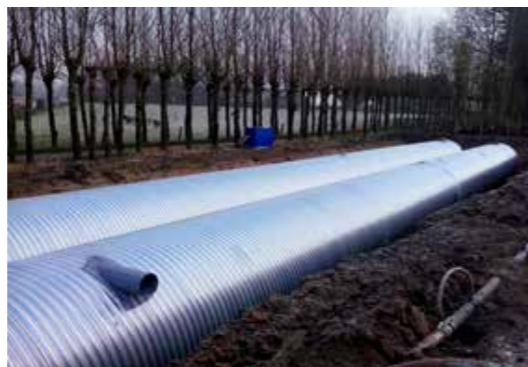
Installation of a rainwater tank
