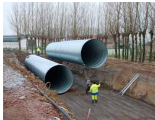
Installation of a rainwater tank
